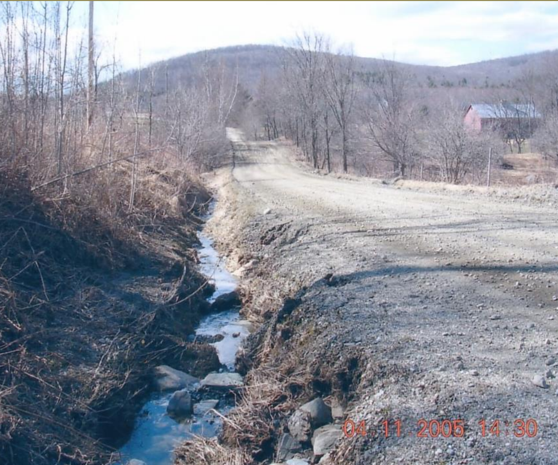
Eroding roadside ditch
