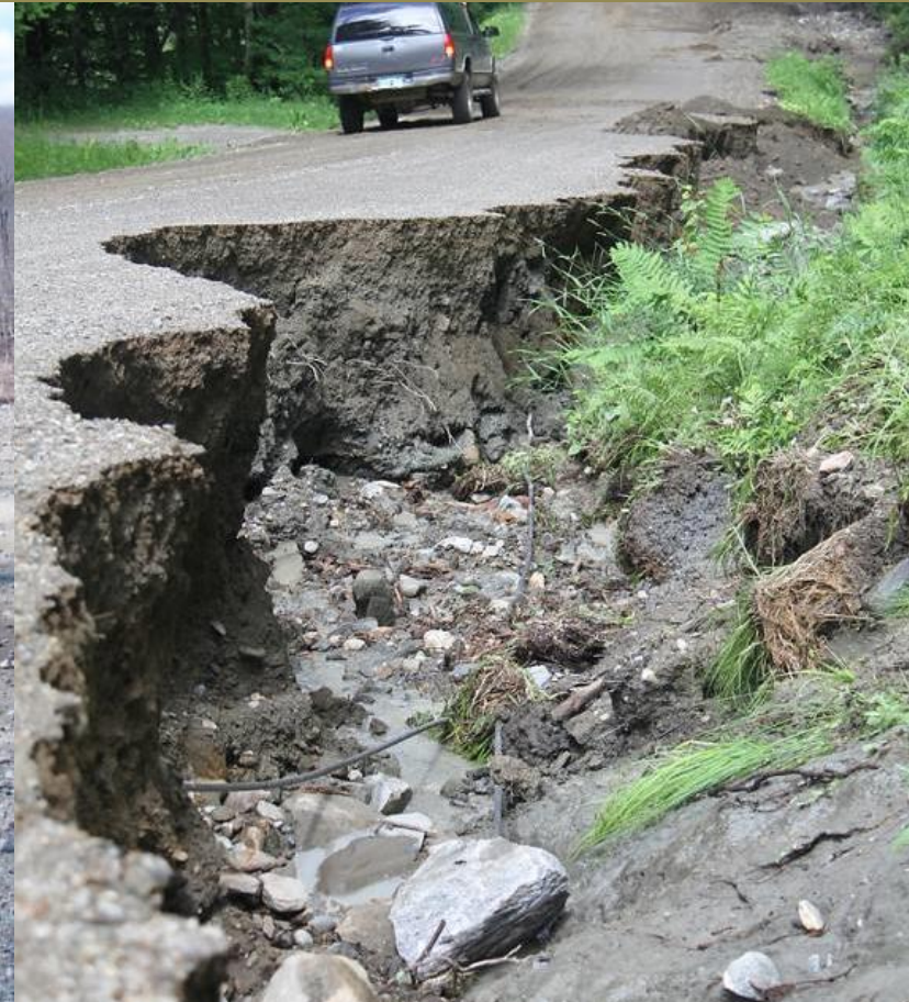
Storm-damaged gravel road
